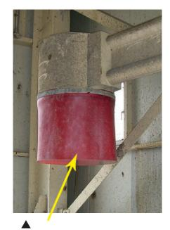
A PUCEST discharge hose: At this mixing plant a PUCEST discharge hose was installed at the swivel arm for "selfcollectors".
